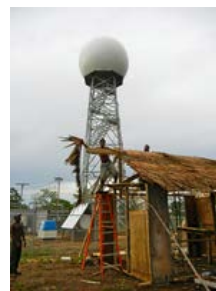
C-band scanning ARM precipitation radar on Manus Island, Papua New Guinea.
