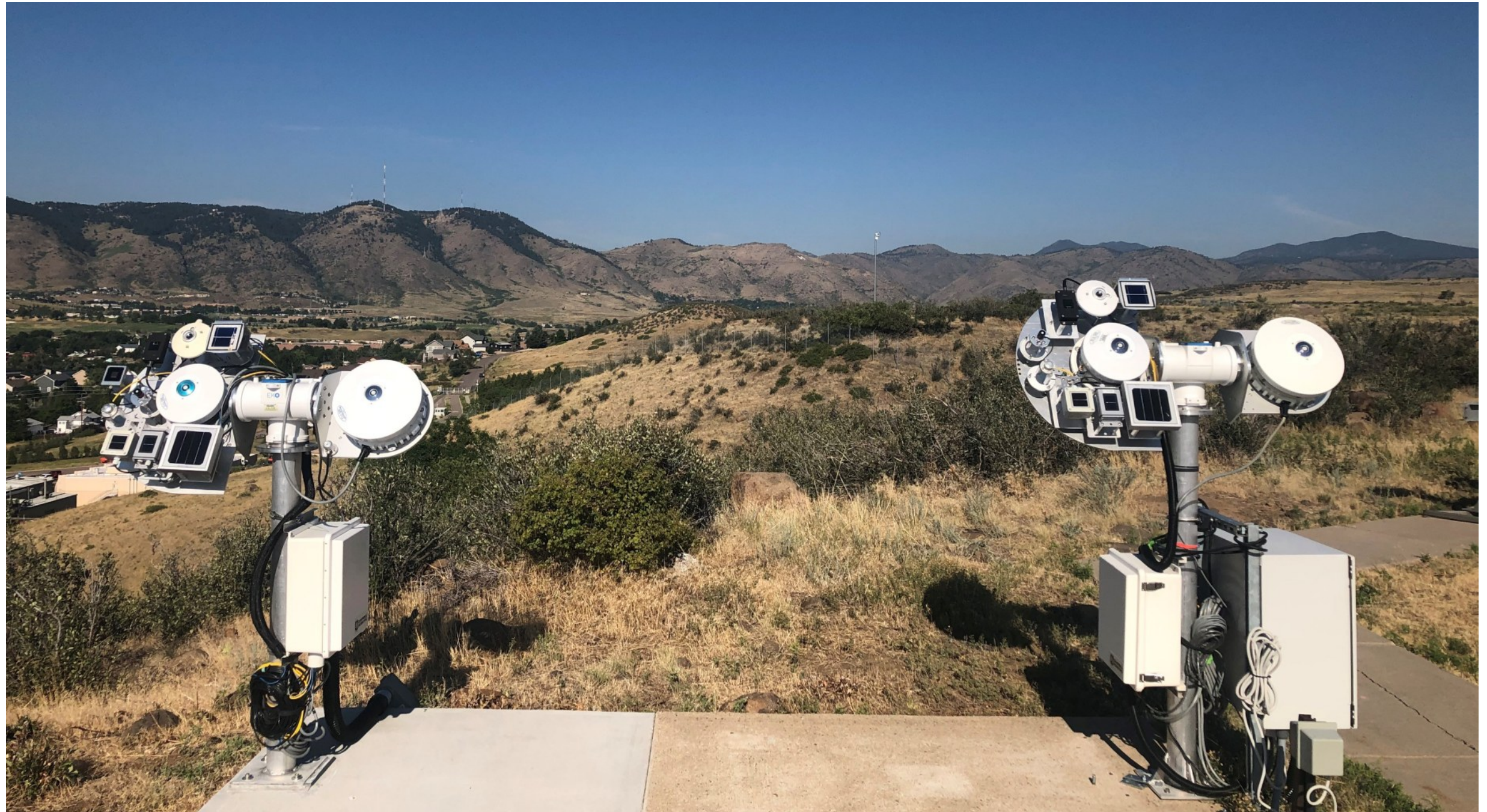
2 and 1-axis tracking WISER – Installed Jan 2020 & Oct 2017
